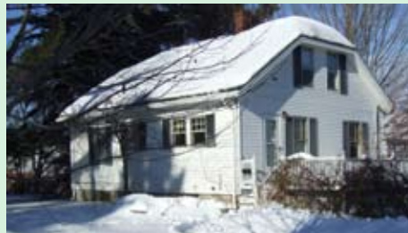
This is the Green Bean on its original foundation on Cross Street in Freeport. Donated by L.L. Bean in 2008, this 1930’s cape was deconstructed and later moved only minutes away to its lot on West Street gifted to Habitat by the Town of Freeport.
